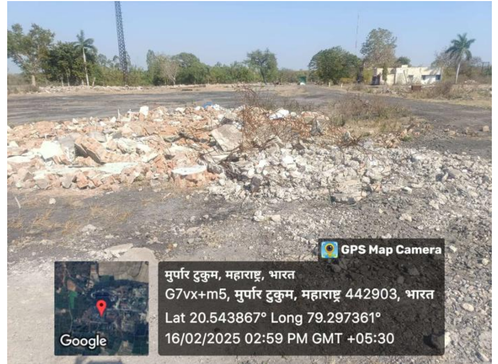
Dismantled Old Weigh Bridge
