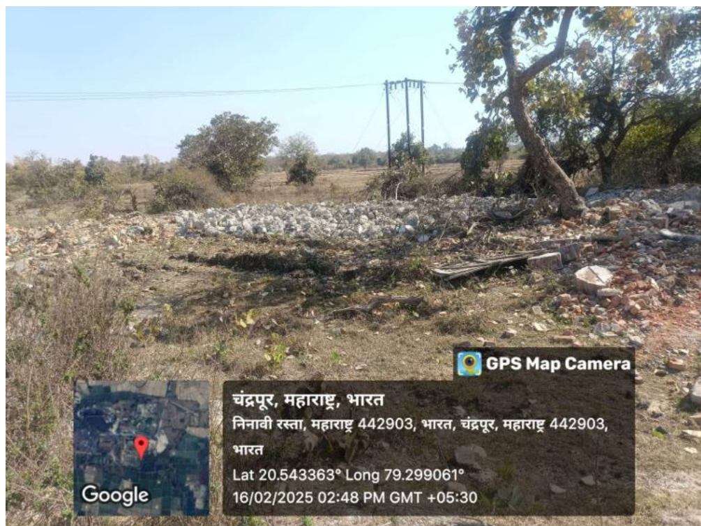
Dismantled Pump House
