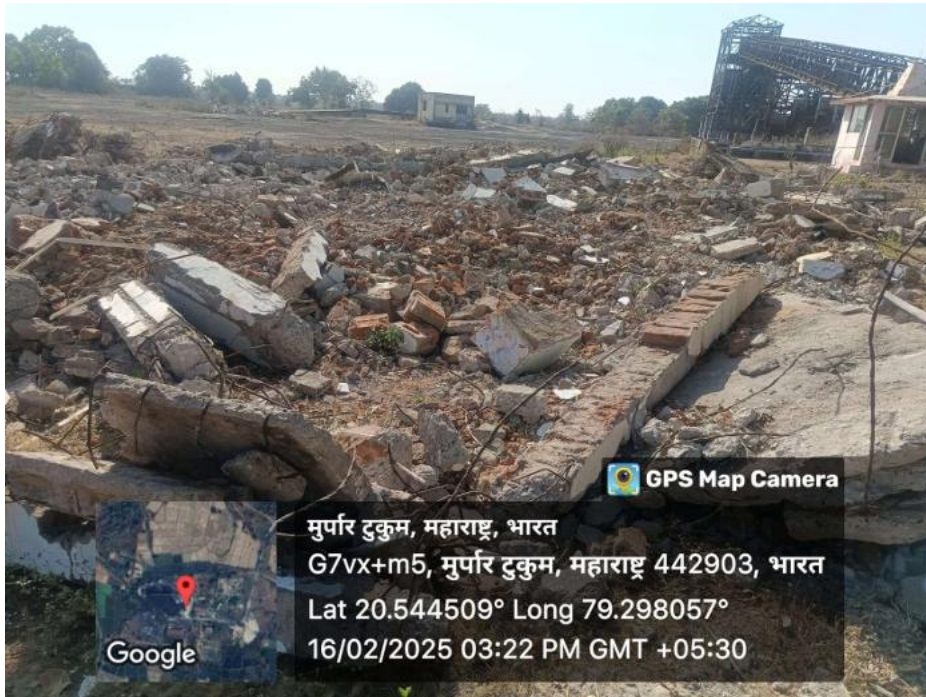
Dismantled Lamp Room
