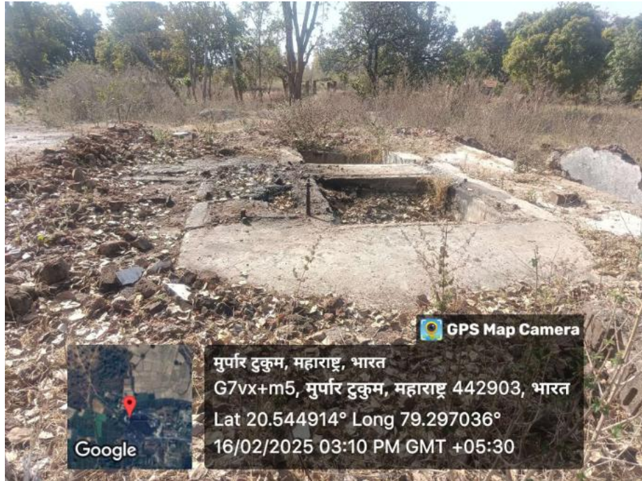
Dismantled Mine Haulage
