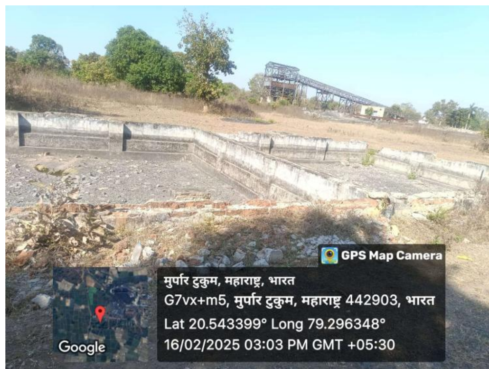
Abandoned Sedimentation Tank / Water filter
