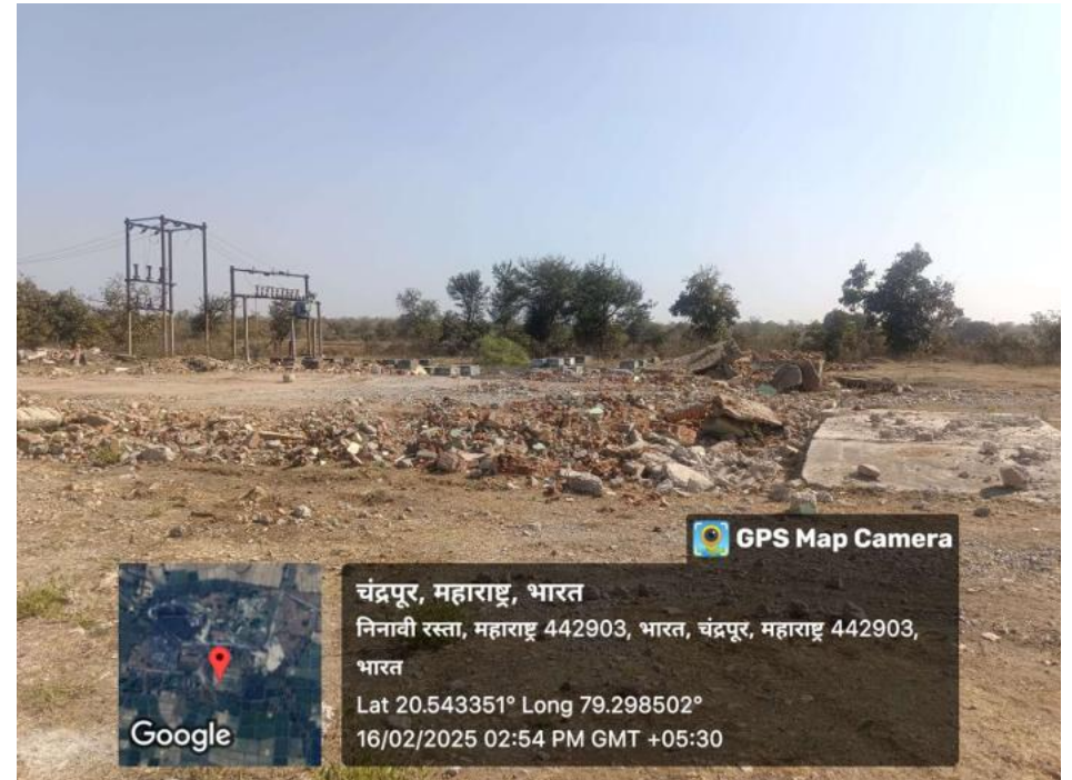
Dismantled Sub Station
