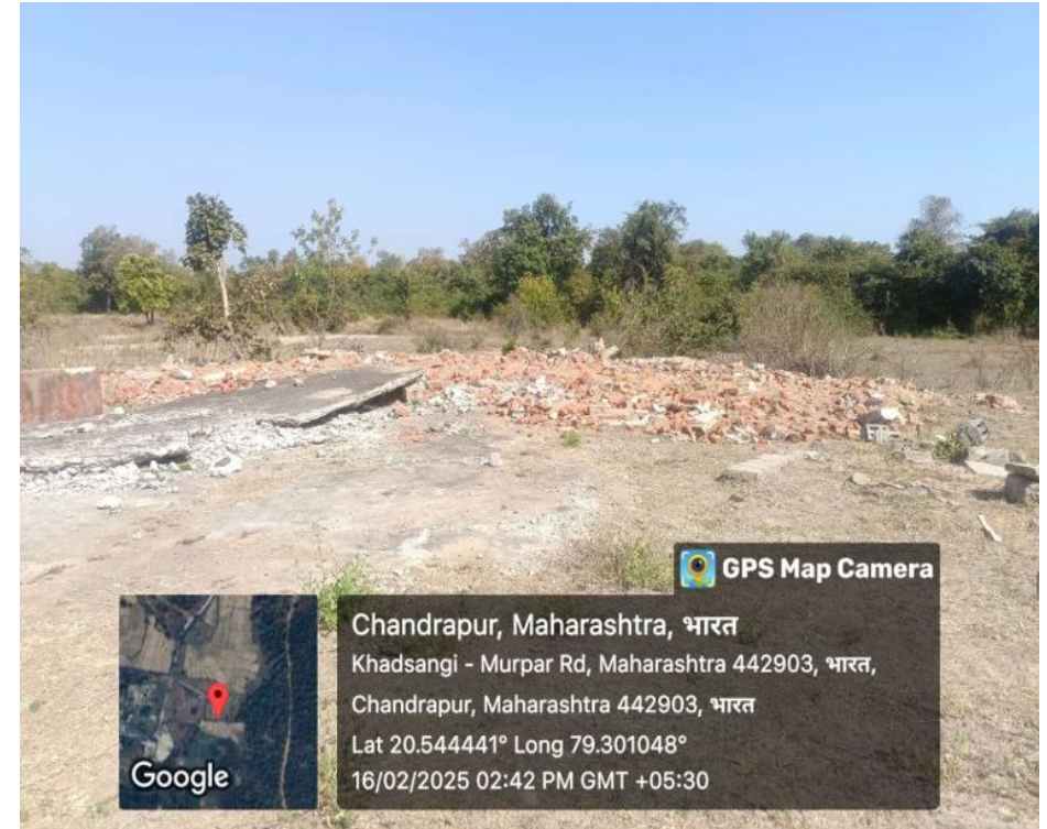
Dismantled Magazine Room
