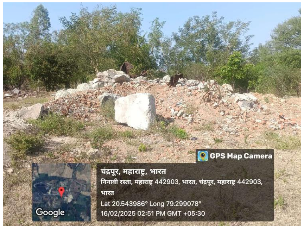
Dismantled Fan house / shaft
