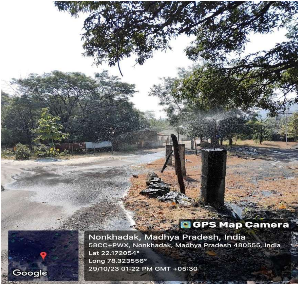
Fixed Sprinklers around coal stockyard and along coal transport road
